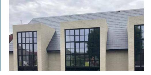
ODC Metro range glazing bars are made from the same material as the main window or sliding system frame, maintaining appropriate proportions. The glazing bars are applied to the sealed glazed panes ensuring U-Values and weather performance remain unchanged.
